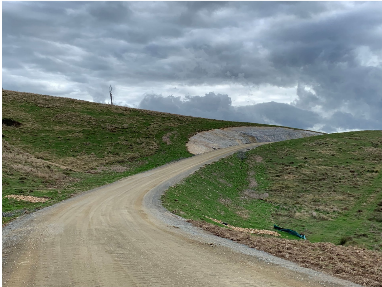
Completed wind farm access track and rehab
