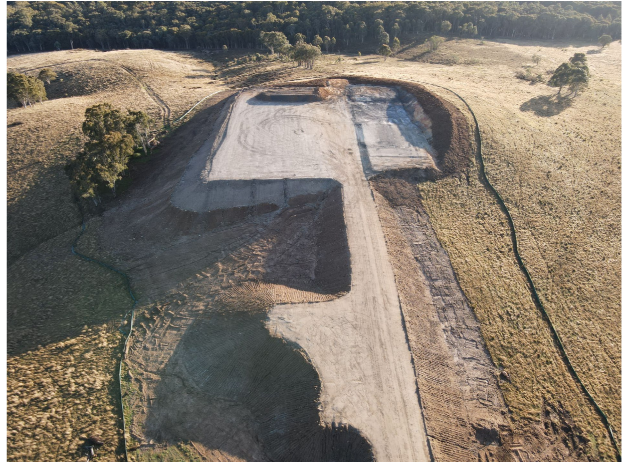
WTG hardstand construction
