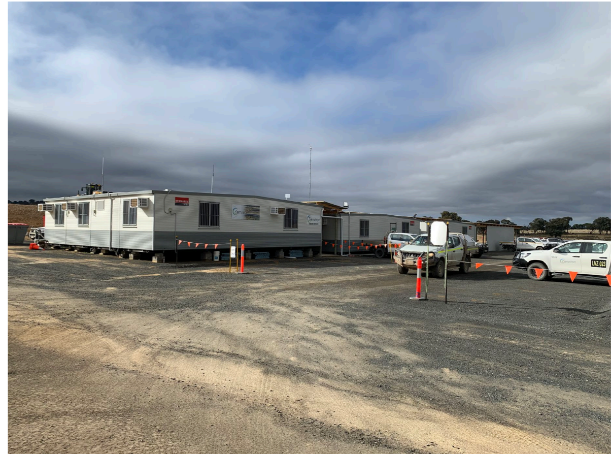
Temporary site office occupied by project staff
