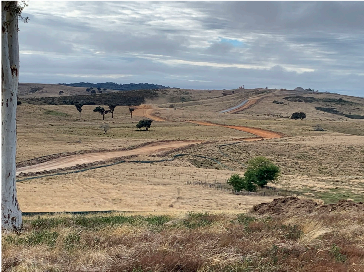
Wind farm access track construction
