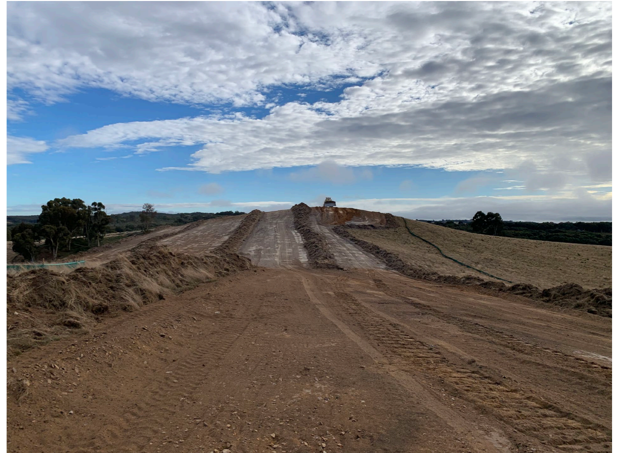
Construction commenced on WTG A12 hardstand
