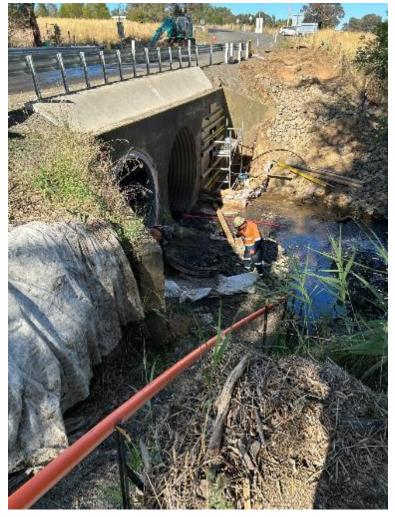
Photo 14: Environmental protection measures at Grassy Creek Road culvert relining
