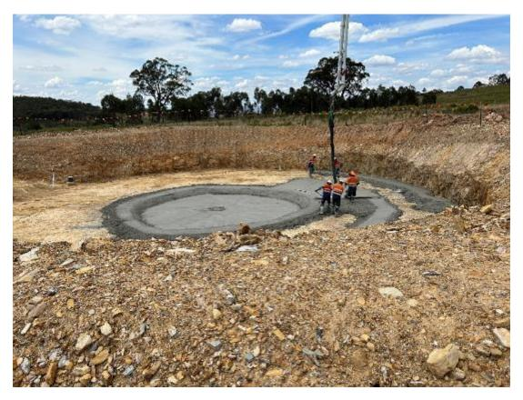
Photo 21: Footing concreting
