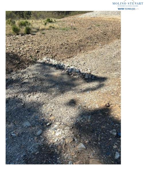
Photo 2: Road drain with rock check dam partly silted up and breached and ineffective.
