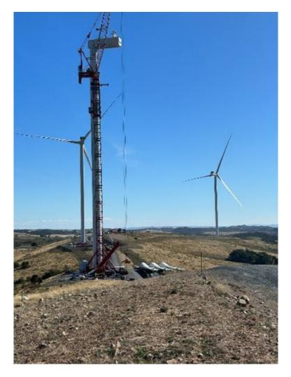
Photo 17: Turbine delivery and erection
