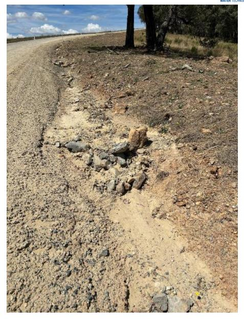
Photo 3: Road drain with rock check dam bypassed and ineffective
