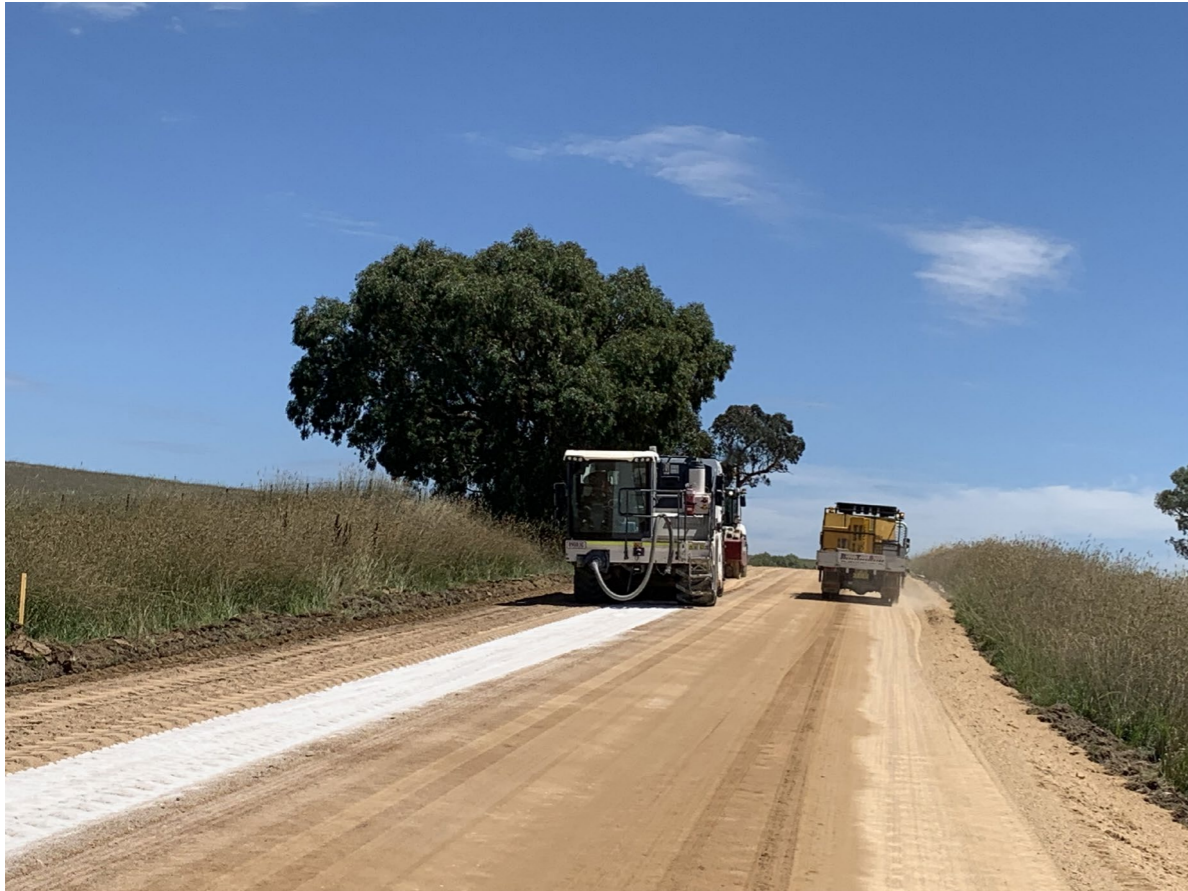
Lime stabilisation of Boorowa-Rye Park road
