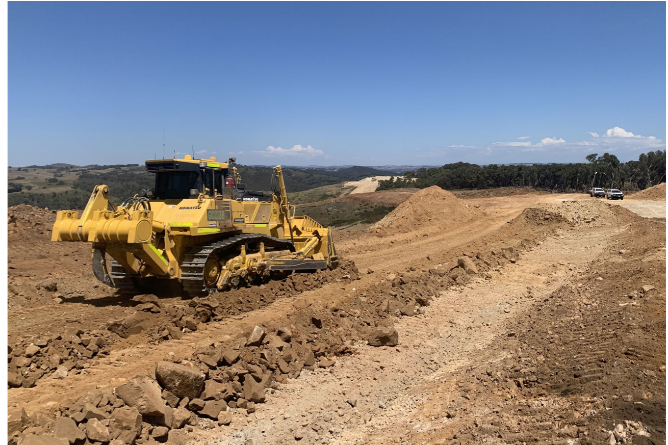
Dozer working on access track formation in northern area
