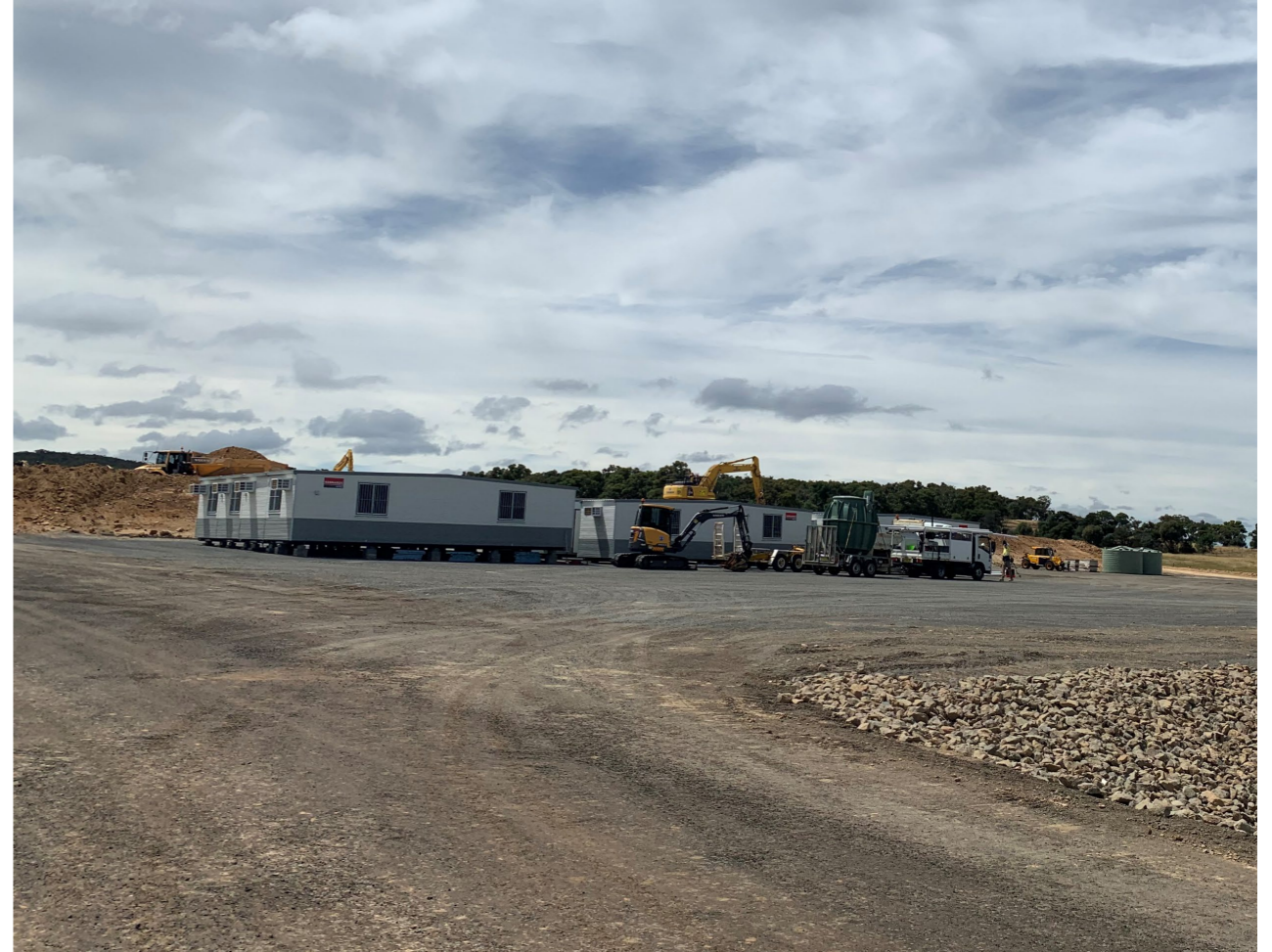
Site office being dropped at temporary compound
