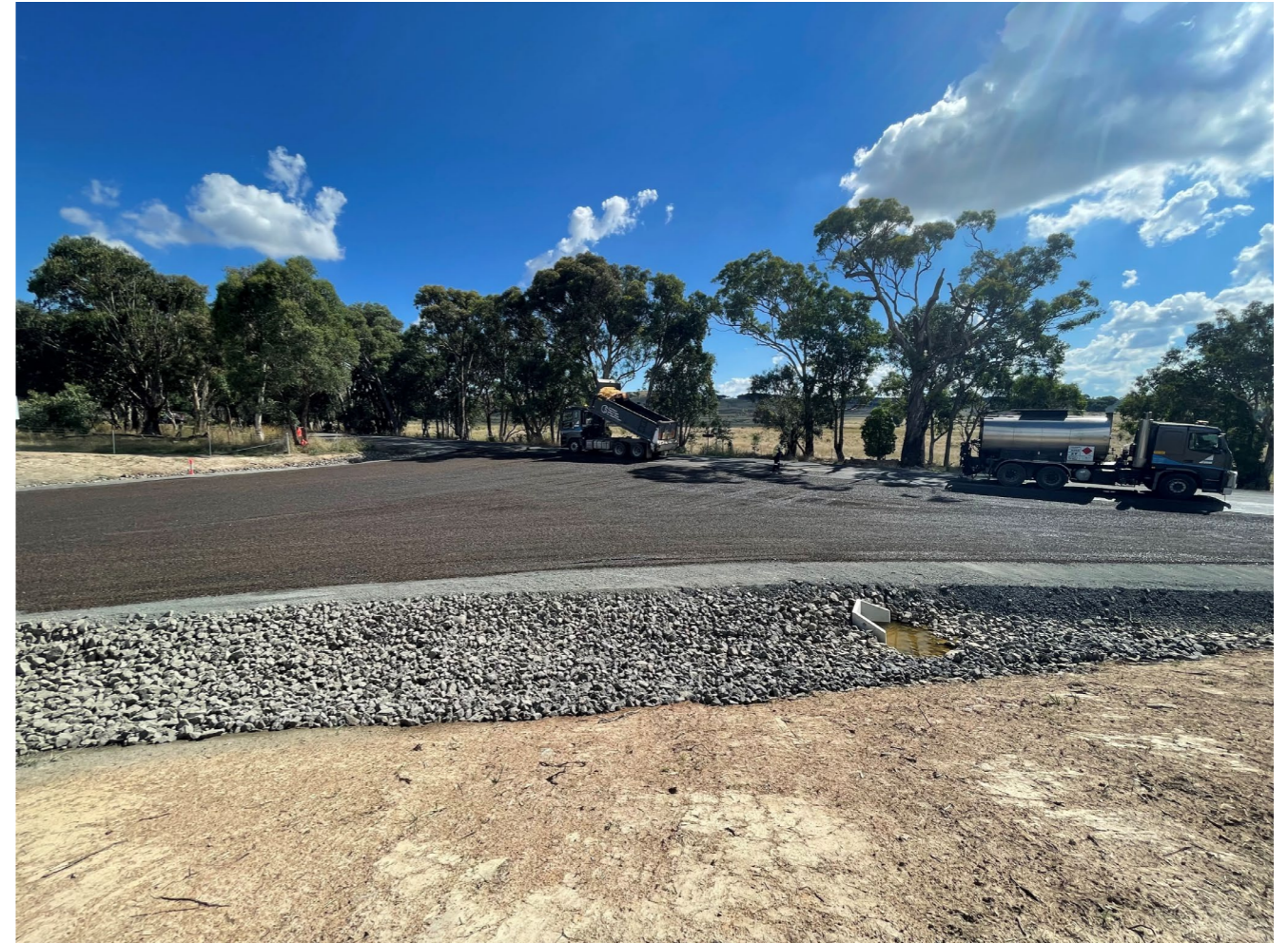
Wind Farm main entry being sealed
