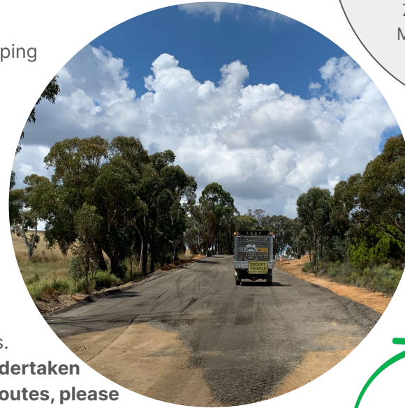
Image: Gravel sheeting of Grassy Creek Road
