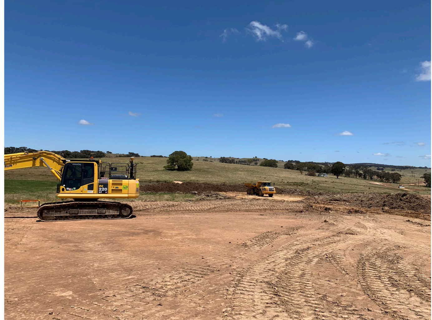
Earthworks commenced on temporary site compound
