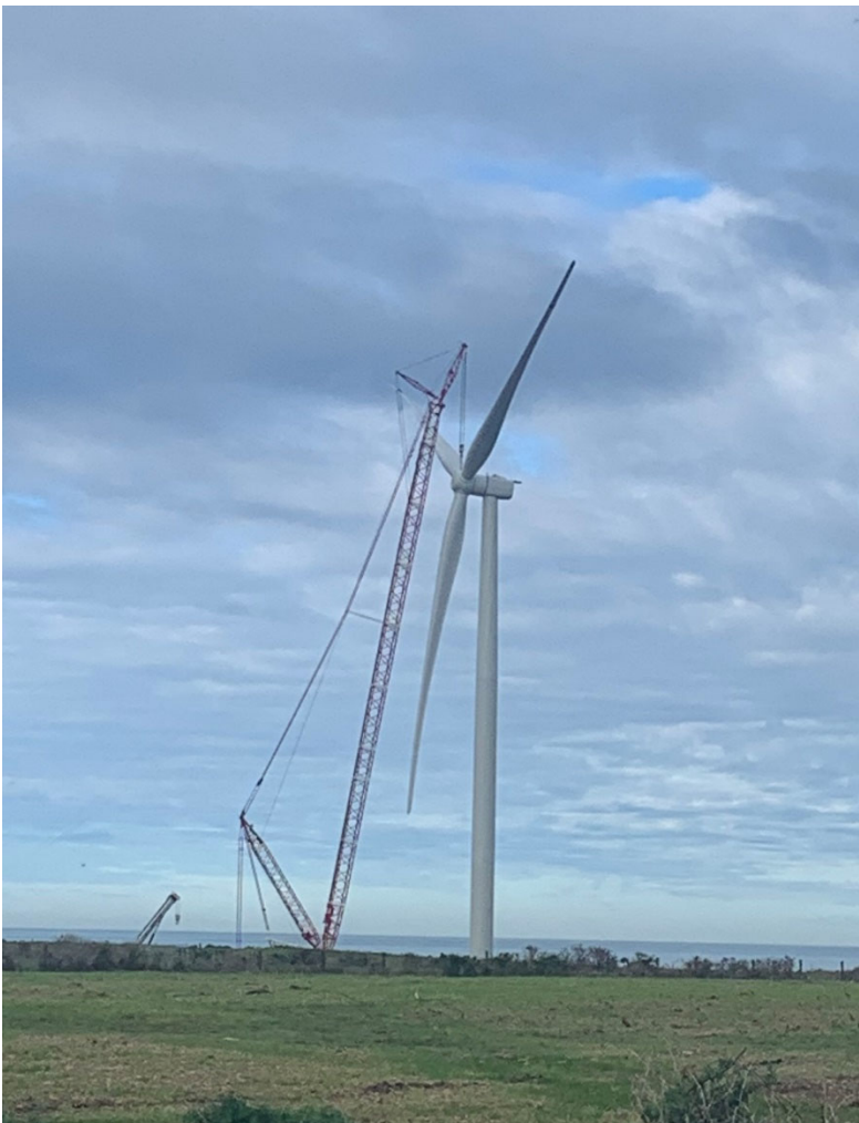
The first turbine at Waipipi Wind Farm
