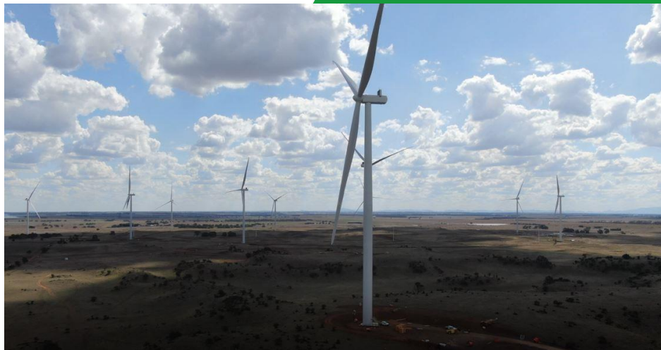
From the first turbine installed to first generation
