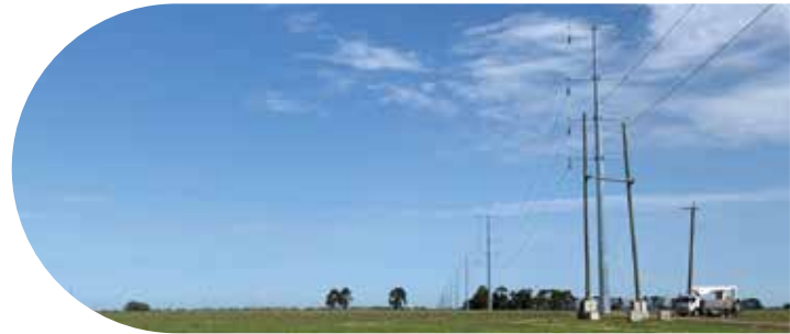
Stringing of transmission line along Castle-Carey Road
