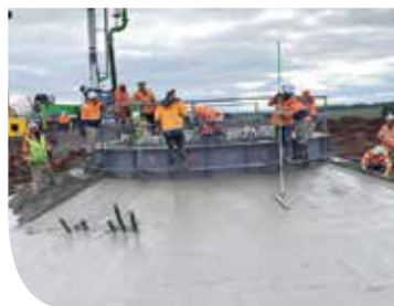
Turbine foundation being poured.
