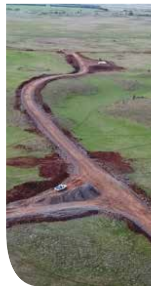
Aerial view of wind farm access track network progress
