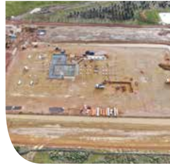
Aerial view of Blue Gums Substation progress.
