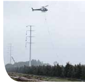
Helicopter stringing the transmission line near the Blue Gums Substation.
