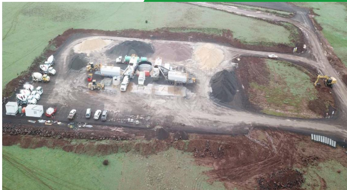
Concrete batch plant
