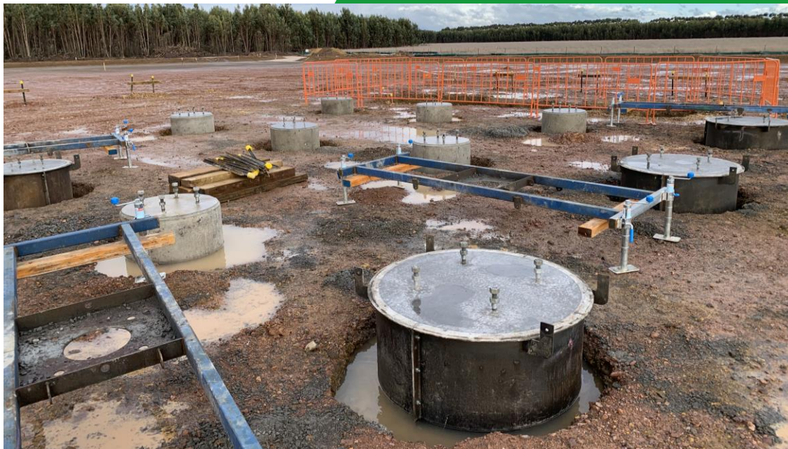
Bored Pile Foundation at Blue Gums Substation
