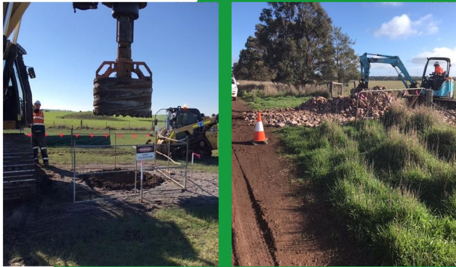
Foundation excavation (L) & Access tracks formation (R)
