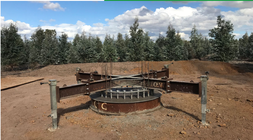
Transmission Pole foundation poured
