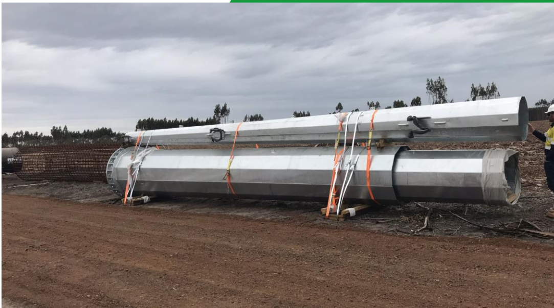
Transmission Line poles arriving on-site
