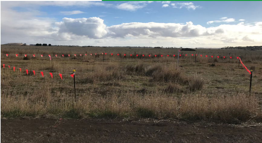
Marked off work areas along Castle Carey Rd
