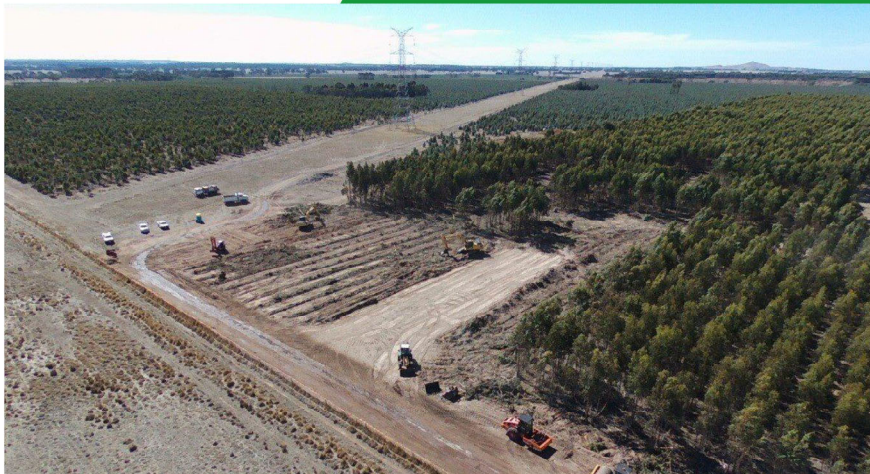
Earthworks and clearing for Blue Gums Substation
