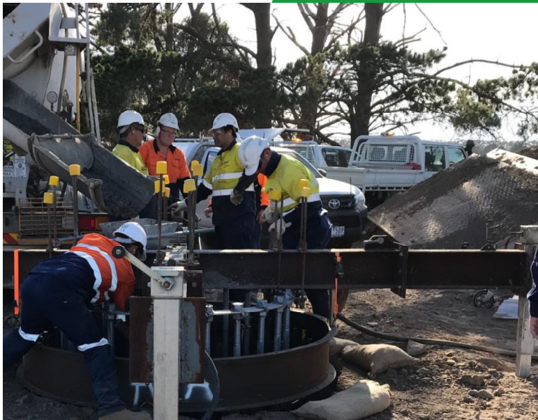
Working on transmission pole foundations
