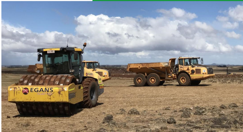
Heavy machinery arriving on site
