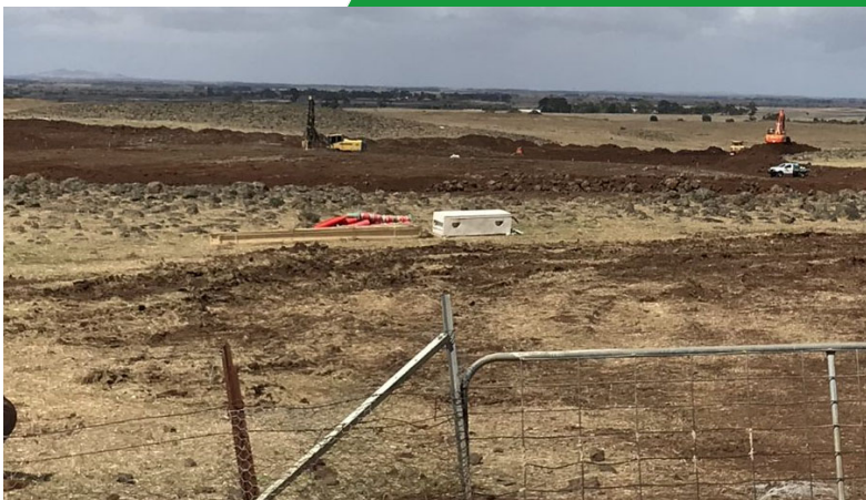
Quarry drilling equipment on site
