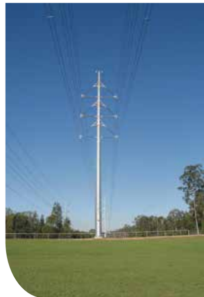
Above: Indicative double circuit steel pole
