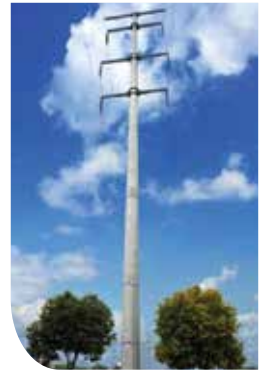
Above: Indicative double circuit steel pole
