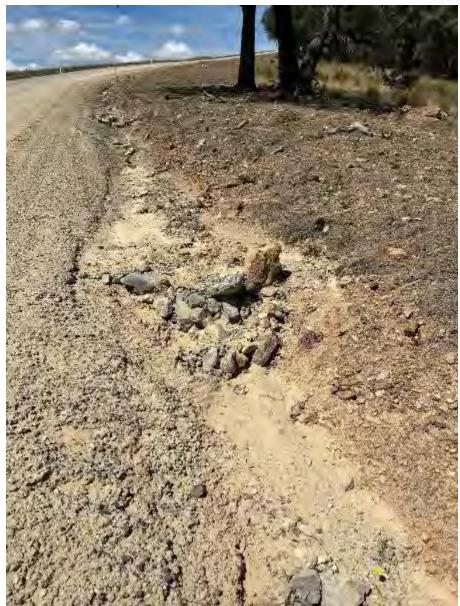
Photo 3: Road drain with rock check dam bypassed and ineffective
