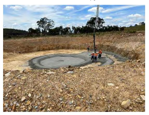
Photo 21: Footing concreting
