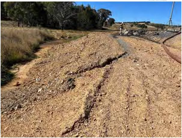
Photo 5: Erosion caused by spillage from a standpipe at the northern batching plant
