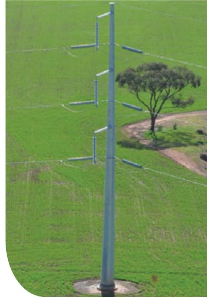
Above: Indicative single circuit steel strain pole 30m
