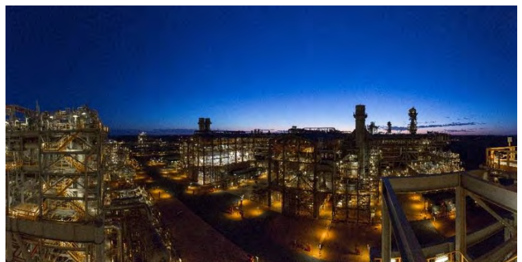
Figure 6 Liquefied natural gas plant on Barrow Island. Photo: Chevron Australia.
