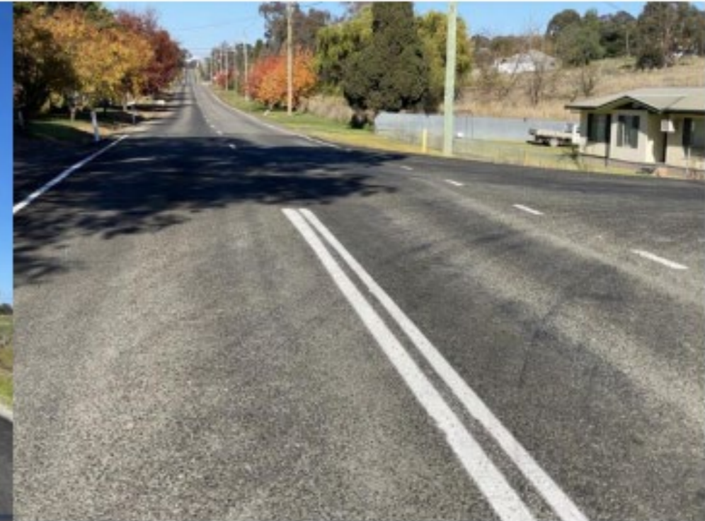
Completed Yass Street / Boorowa Road intersection
