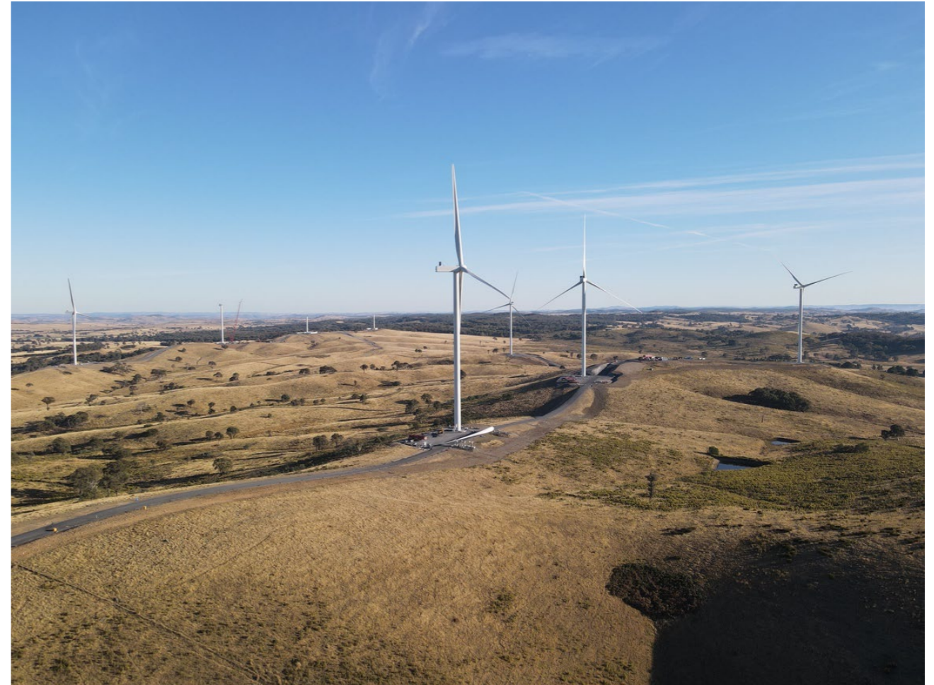
WTG A07 looking north
