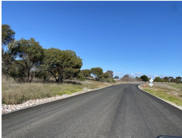
Figure 2: Resealed Trucking Yard Road
