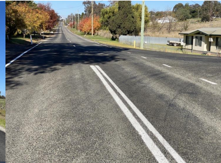
Figure 3: Completed Yass Street / Boorowa Road intersection
