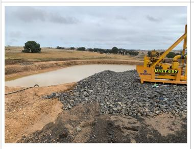
Photo 11: Sediment basin (water re-used for dust suppression)
