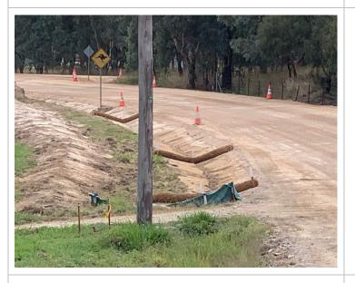
Photo 7: Erosion and sediment control, progressive installation
