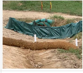
Photo 6: Erosion and Sediment Control, drainage protection
