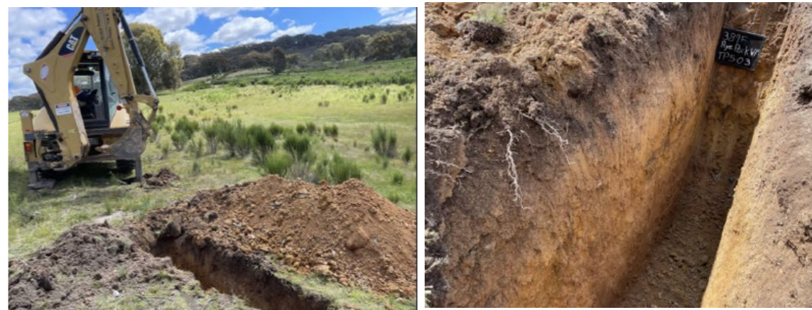
Example Test Pit - Rye Park Wind Farm
