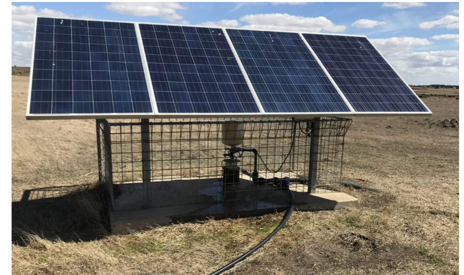
Example Solar Powered Water Bore – Dundonnell Wind Farm
