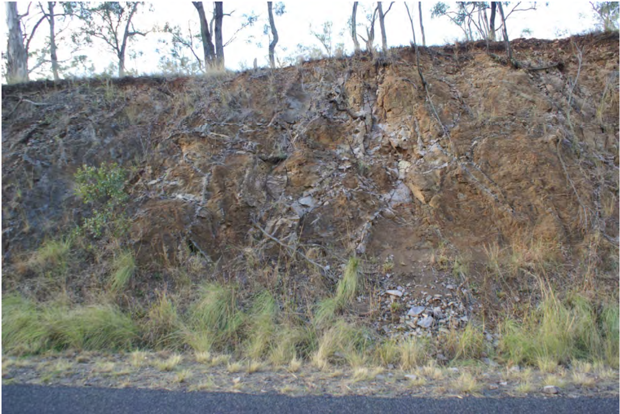
Figure 5.3. View of South Western Side of Road Cutting
