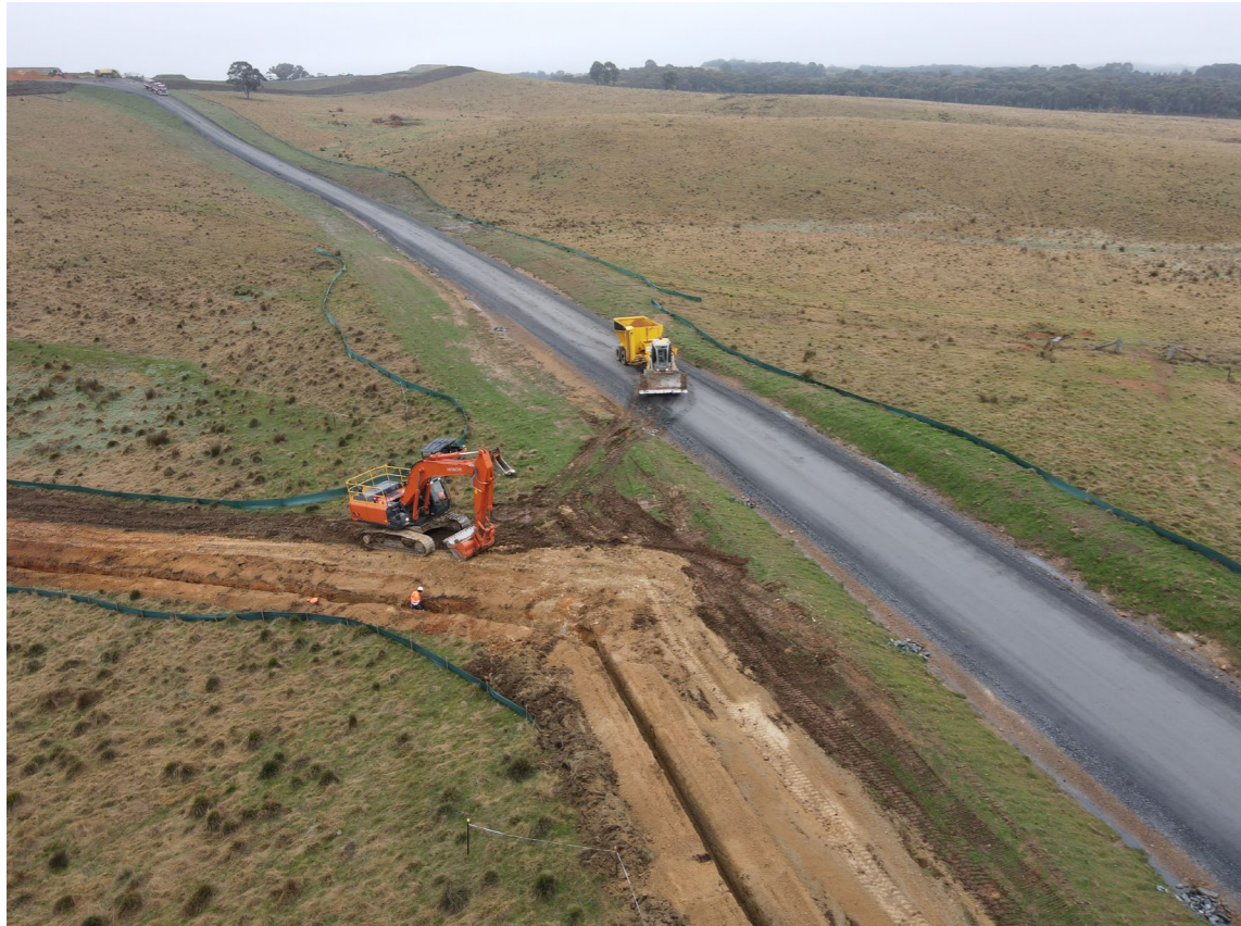
Underground cable trenching commenced
