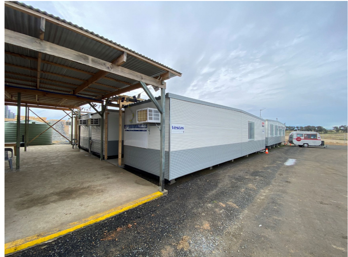
Temporary site office stage 2
