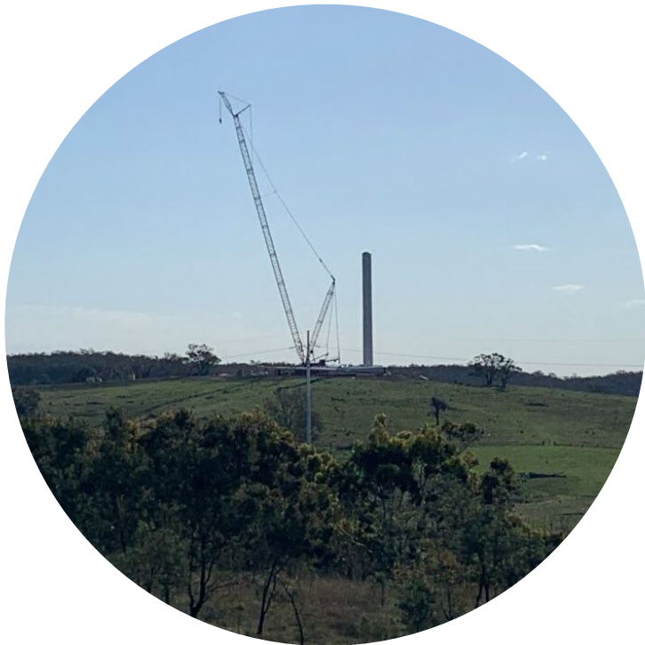
Figure 4: Assembling the tower
