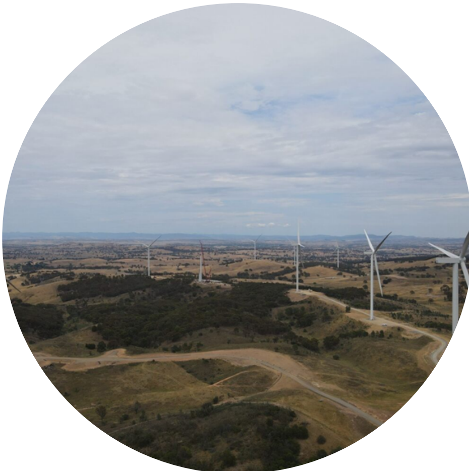
Figure 2: View from turbine G03
