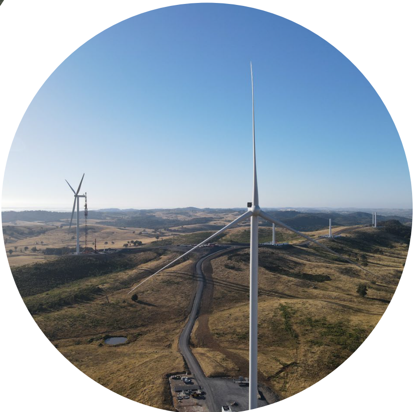
Figure 5: The first generating turbine
