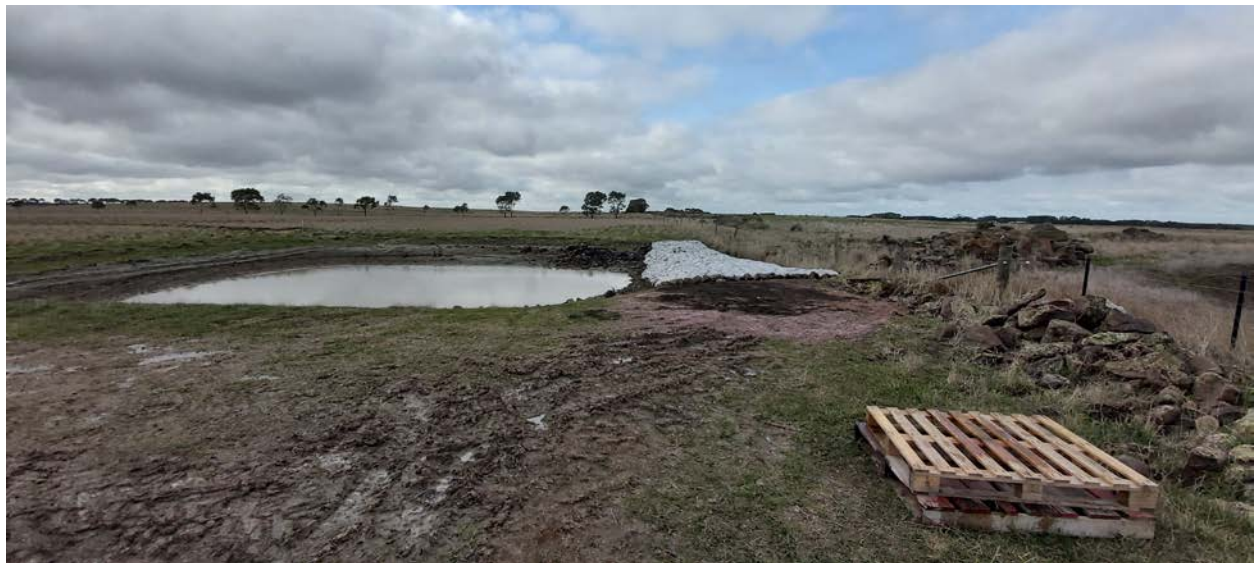
Photo 2. Finished sandbagging at wetland drain.
