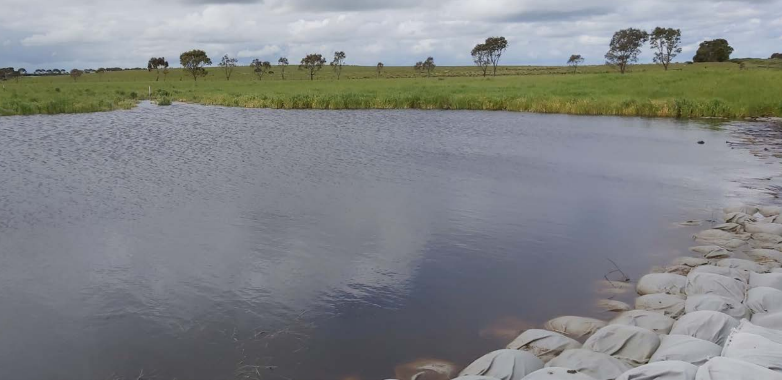
Photo 1. DUN001 Wetland with the geo-fabric sandbags installed (October 2022)
