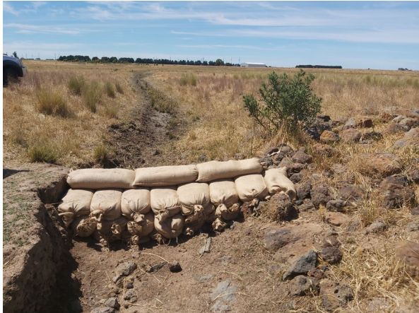
Photo 7. Sandbags placed in drain
