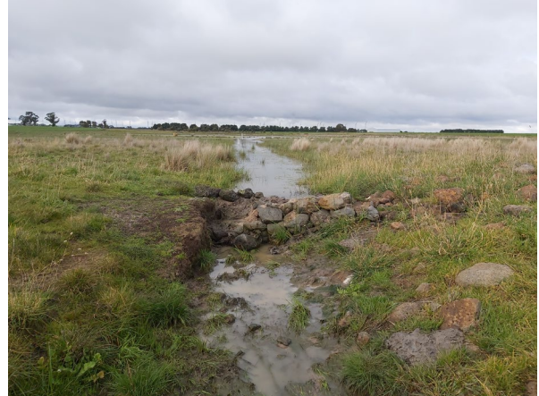
Photo 8. Sandbags starting to degrade (July 2021)
