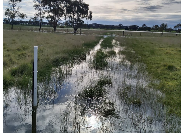
Photo 15. Water level over sandbags within the drain (August 2021)
