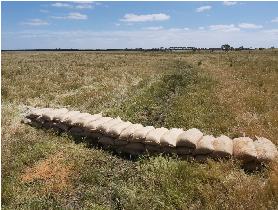
DUN-BCP-001 – Temporary measures employed, sandbag block in drain 10/12/2020
