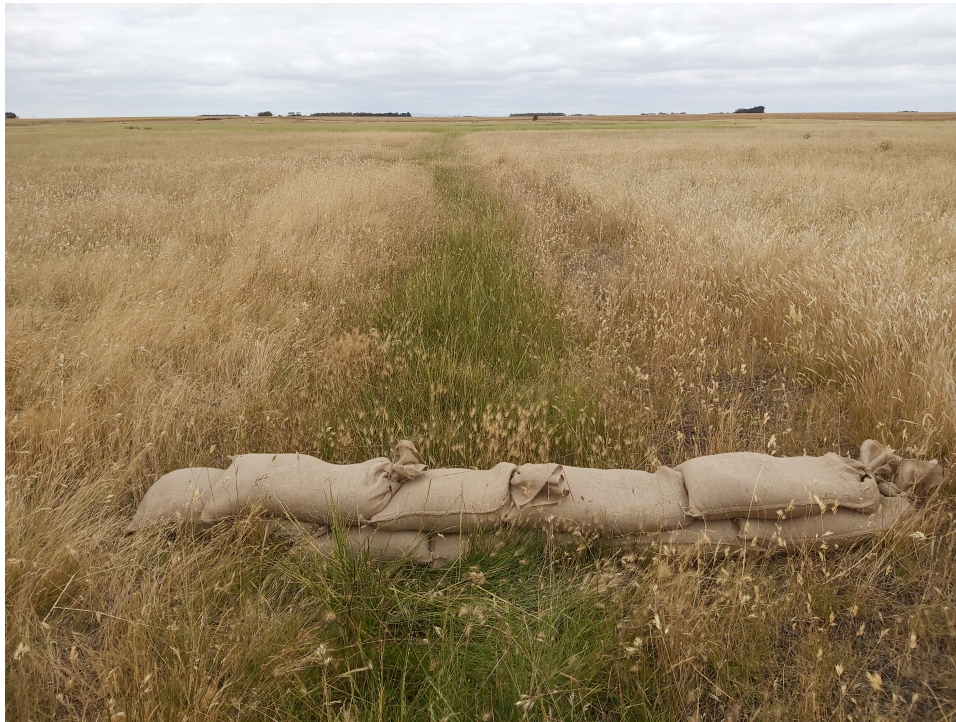
DUN-BCP-004 – Temporary measures employed, sandbag block in drain 08/12/2020
