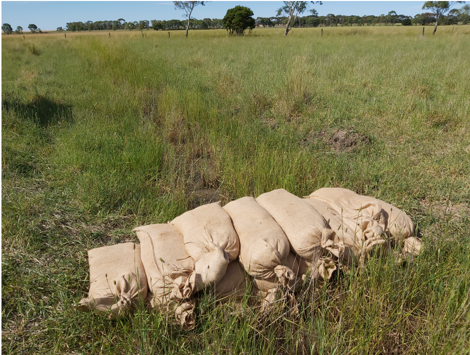
DUN-BCP-003 – Temporary measures employed, sandbag block in drain 30/11/2020
