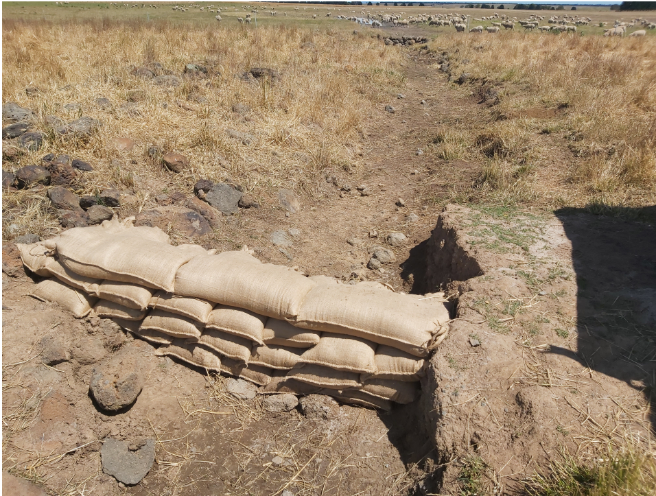
DUN-BCP-002 – Temporary measures employed, sandbag block in drain 30/11/2020
