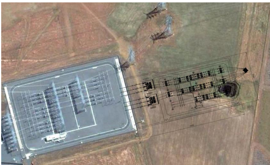
Photograph 2-3 Typical 500/220kV Substation
